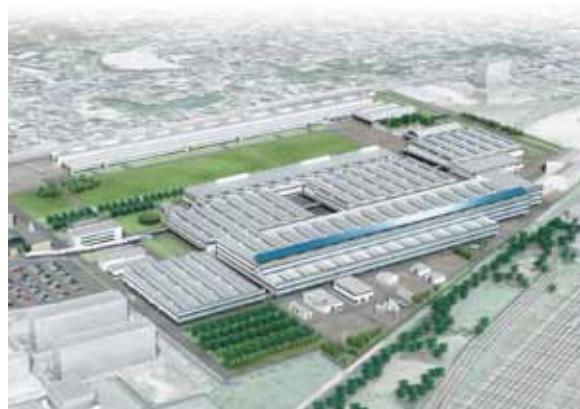
Renovation of the Hamamatsu Workshop (completion image)
