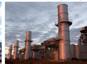
Dampier LM6000 GT 5 x 45 MW (2013)
