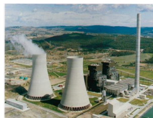
Mt Piper PVC Boiler 2 x 660 MW (1987)
