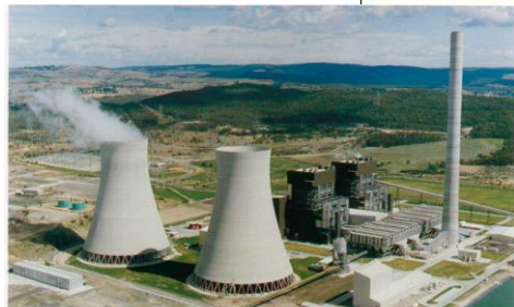
Mt. Piper Power Station (for Energy Australia) 2x660MW (Portland, NSW)
