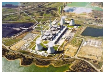
Bayswater PVC Boiler 4 x 660 MW (1986)
