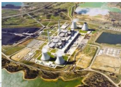
Bayswater Power Station (for AGL Macquarie) 4x660MW (Hunter Valley, NSW)
