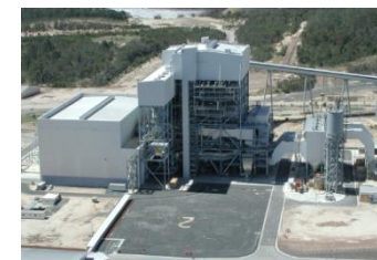
Tarong North SOVR Boiler 1 x 450 MW (2003)
