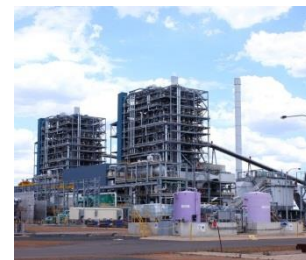
Bluewaters PVC Boiler 2 x 229 MW (2009)
